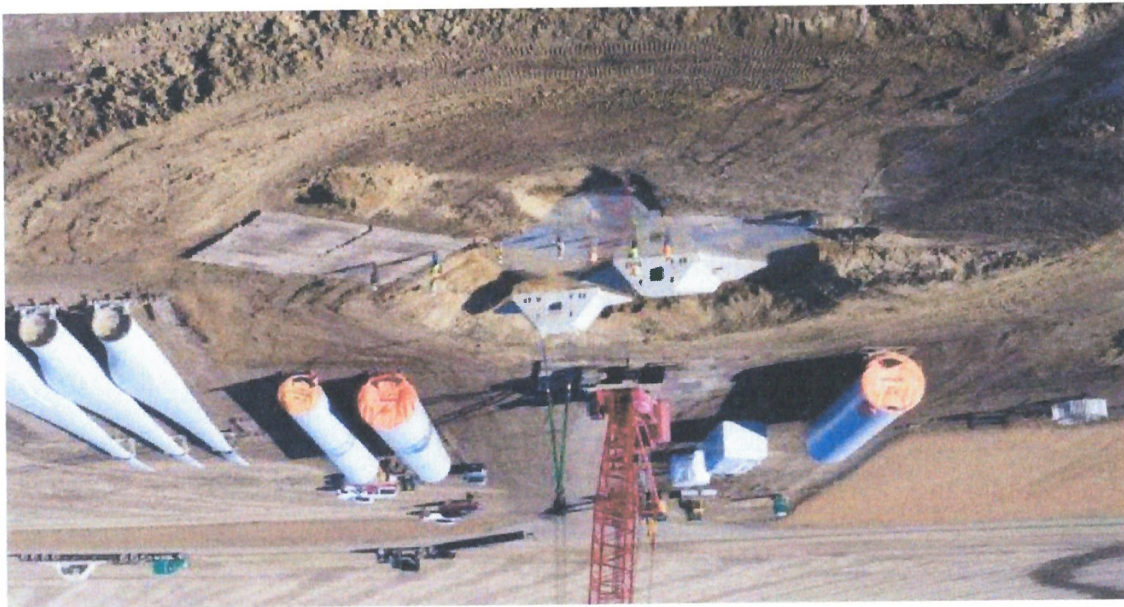
Plate F Scale of turbine base construction pads (4 no. proposed). Note the scale of each of the three BLADES relative to the construction workers.
